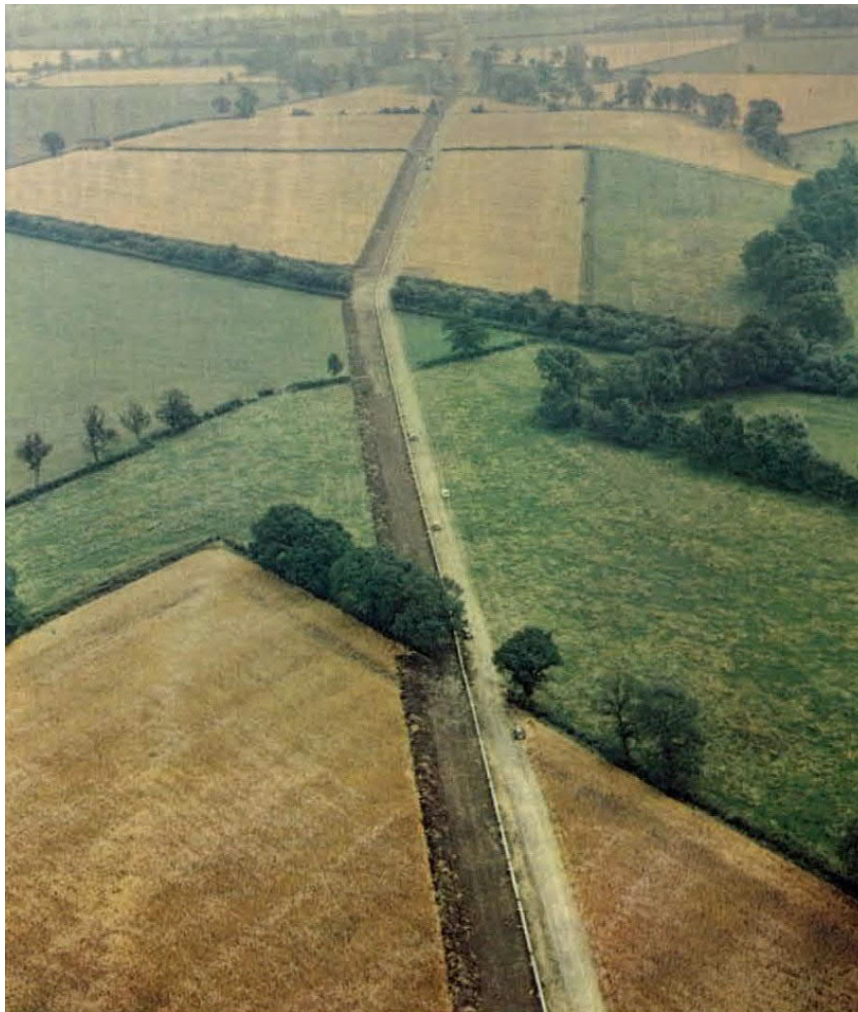
Figure 5.13. The route of the purpose-built pipeline to the Tunnel Cement works at Pitstone in 1972. Source - National Gas Archive.
