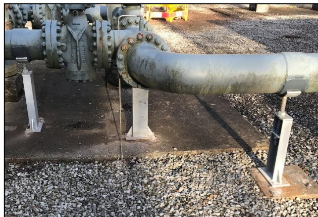
Figure 8 - Following refurbishment, with adjustable support and neoprene insert
