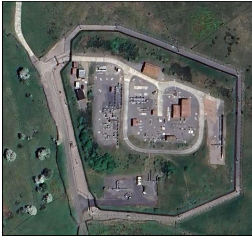
Figure 1 - Aerial view of one of our biggest Offtakes, Dowlais
