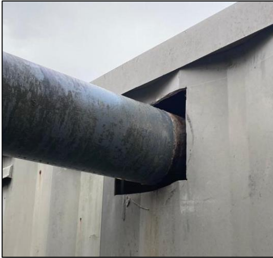
Figure 11 – Original close transition through building wall cut away
