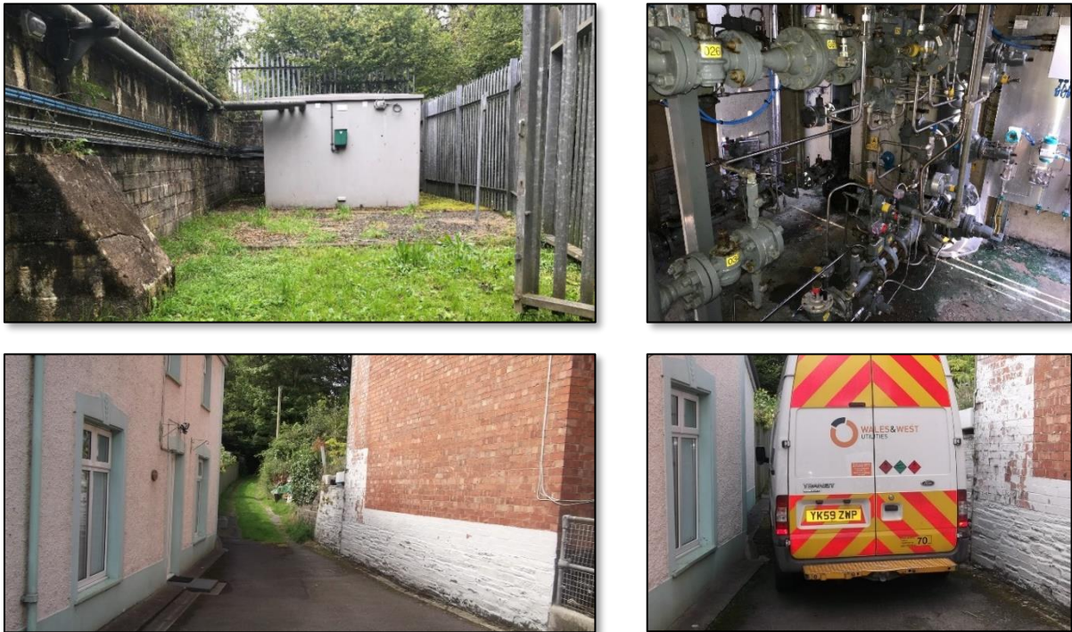
Figure 16 – Top left: old compound, top right: old subsystem, bottom left and right: access to old site
