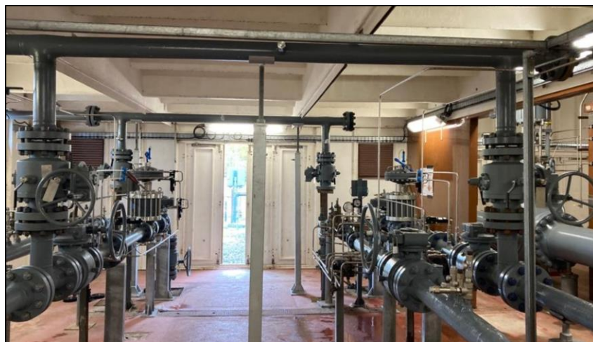
Figure 6 - Example of pressure regulating streams, Dowlais Offtake
