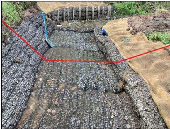
Figure 10 - Completed project showing cleared vegetation and installed rock matting over the pipeline
