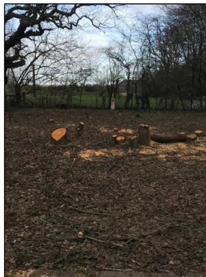
Figure 17 – After: trees that were within 3 meters of the pipeline have now been removed
