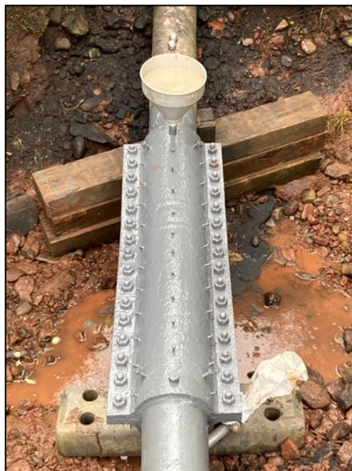
Figure 9 - Pictures showing the newly installed shell (left) and the shell ready to be grout-filled (right)
