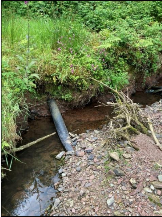
Figure 8 - Pictures showing the exposed pipeline and vegetation growing around the eroded riverbank
