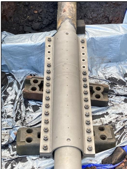
Figure 9 - Pictures showing the newly installed shell (left) and the shell ready to be grout-filled (right)
