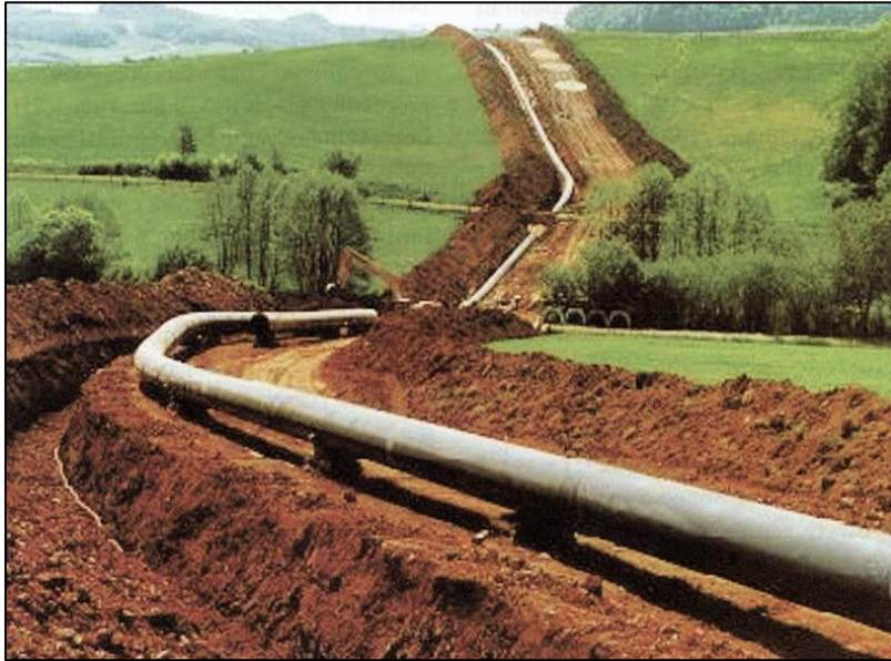
Figure 1 – Cross country pipeline under construction (example photo, taken from: https://www.conservesolution.com/portfolio/cross-country-pipeline-a20-project/ )
