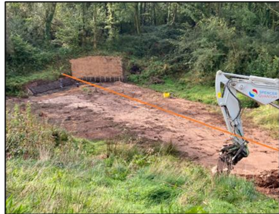
Figure 10 - Completed project showing cleared vegetation and installed rock matting over the pipeline
