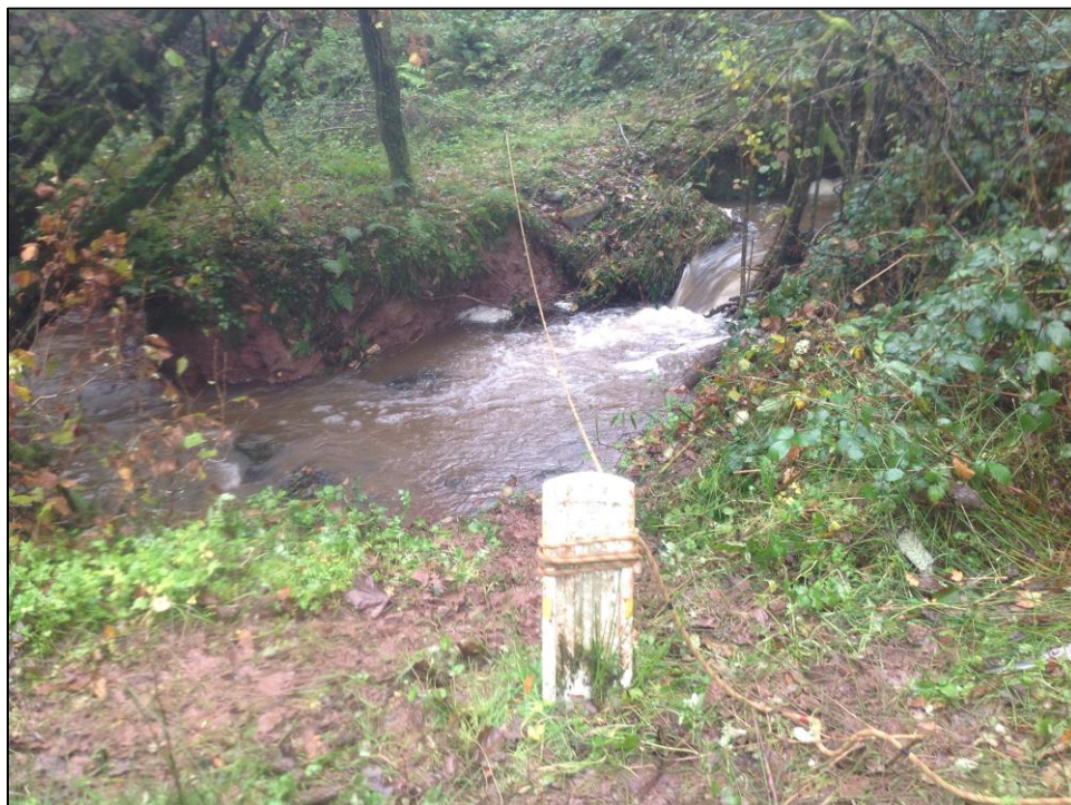
Figure 7 - River in full swell in October where the bank is starting to erode (rope indicates pipeline route)
